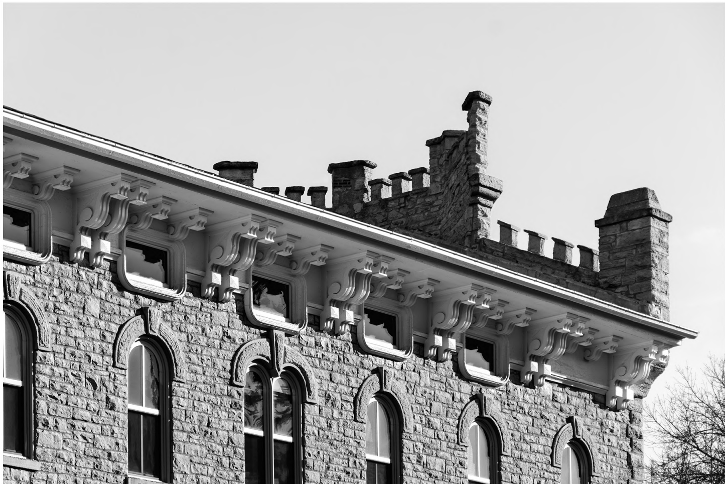
Wheaton College, Blanchard Hall, West Wing and Parapet, 2012
