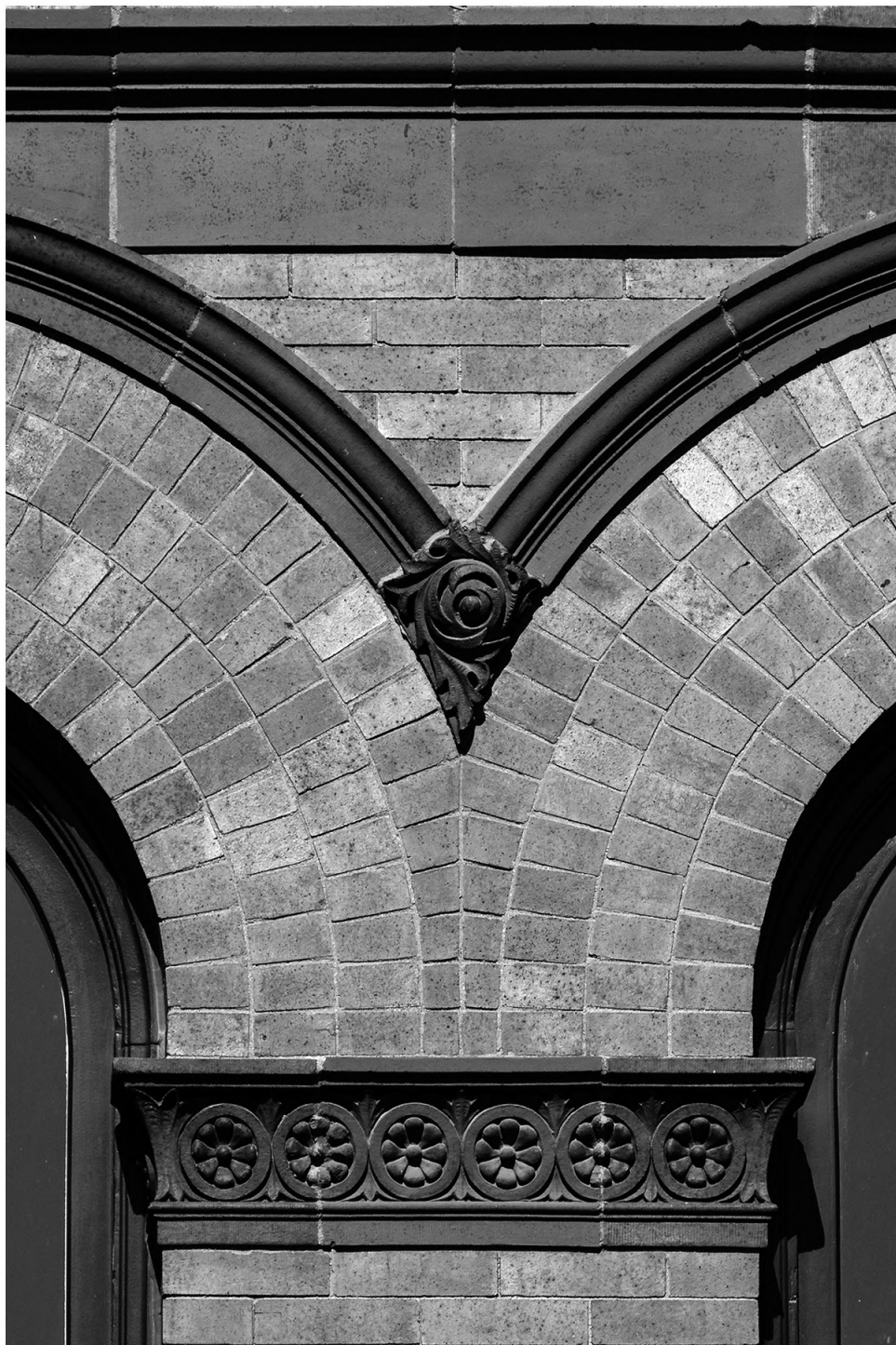
Former DuPage County Courthouse, Wheaton, IL, Romanesque Arch Detail, 2011
