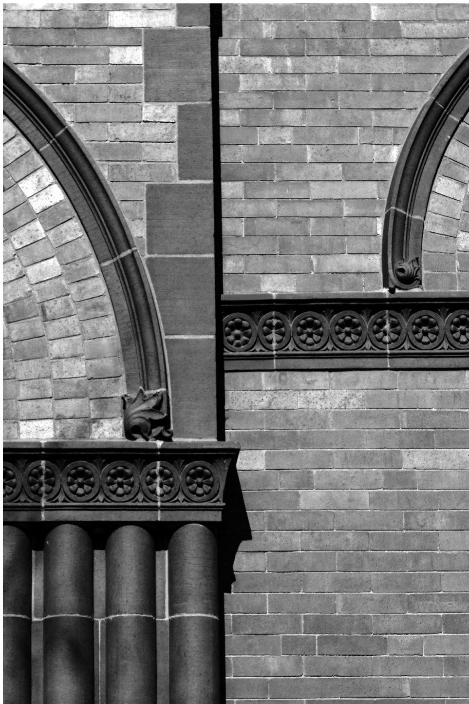
Former DuPage County Courthouse, Wheaton, IL, Wall Details, 2011
