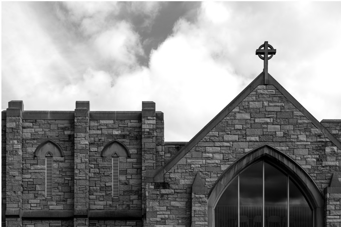
Gary United Methodist Church, Wheaton, IL, West Façade and Parapet, 2021
