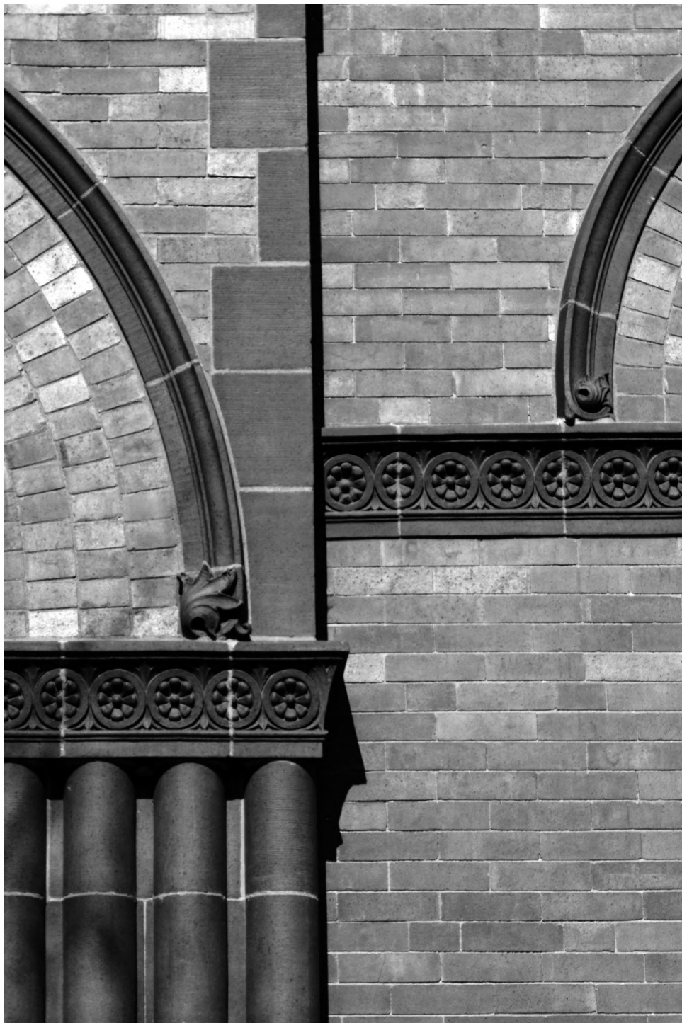
Former DuPage County Courthouse, Wheaton, IL, 1896, Wall Details
