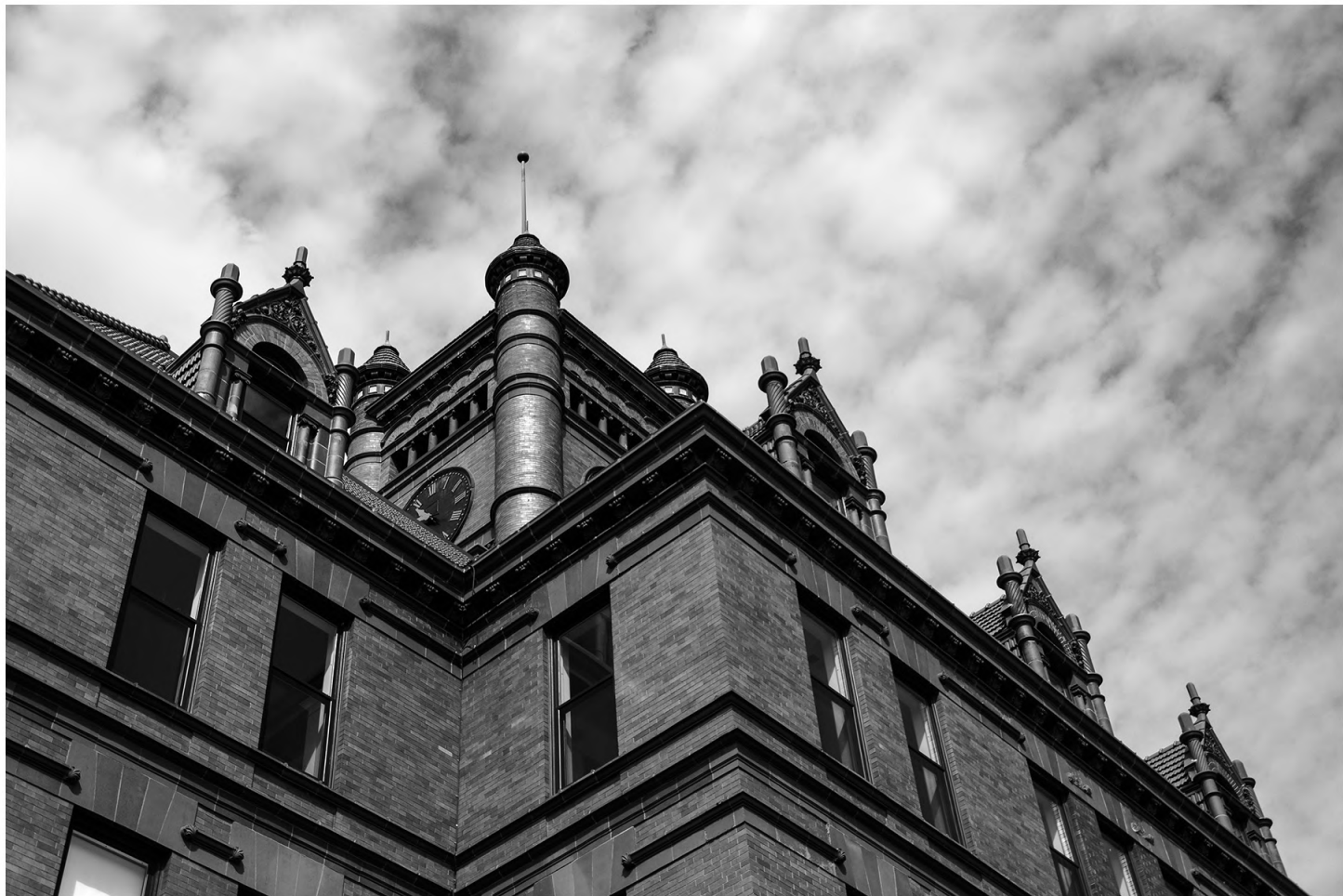
Former DuPage County Courthouse, Wheaton, IL, 1896, View from SE 2011
